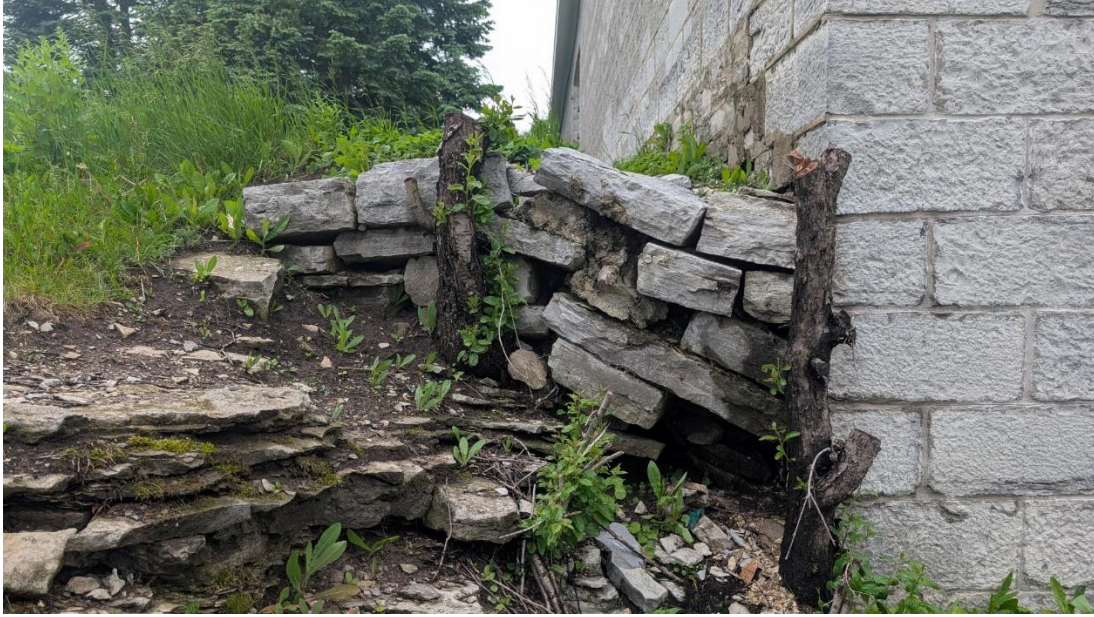
Existing retaining wall along the south-side of the east-end of The Barn.
