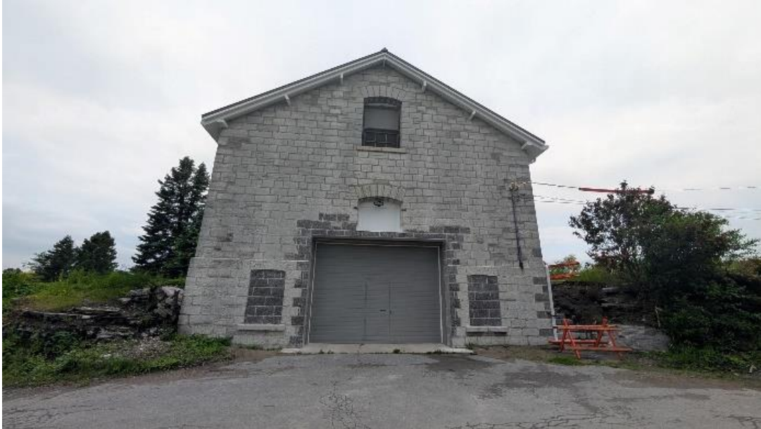
Top Image: View of The Barn's east-end elevation.
