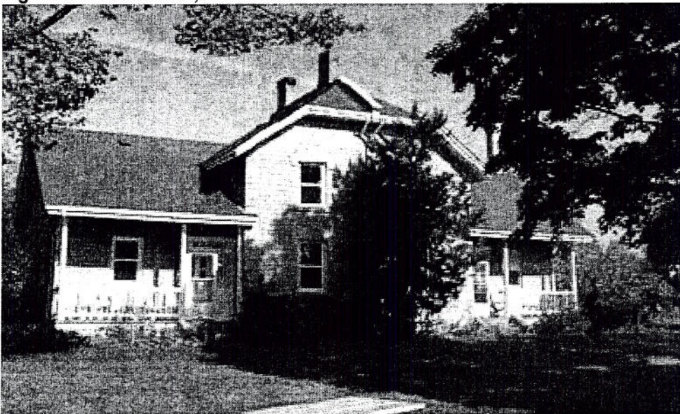
Figure 4: Rodden Park, view of farmhouse.
