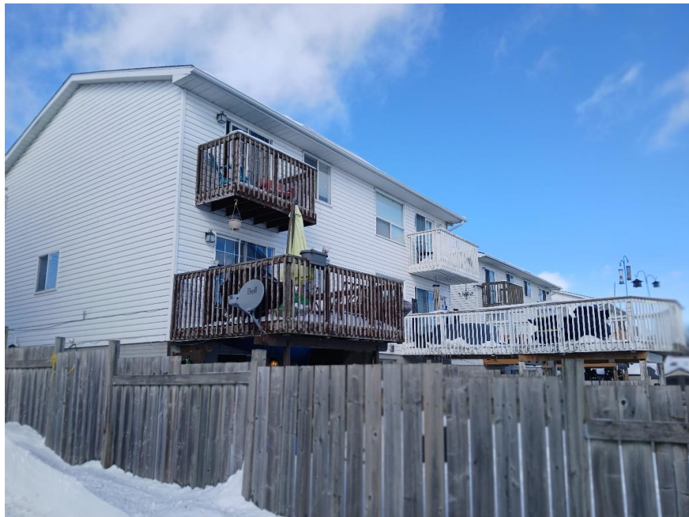
Figure 2: Rear Balconies on Adjacent Properties to the North (1041 and 1043 Montreal St)
