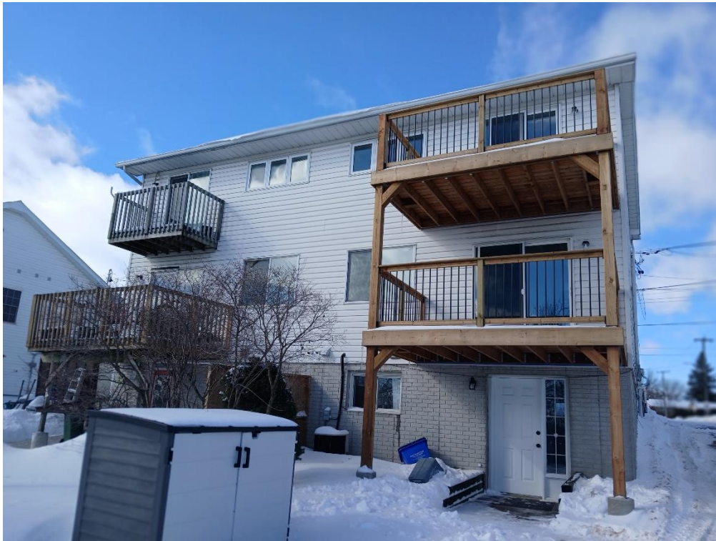
Figure 1: Rear Balcony Expansion (1037 Montreal Street on the Right)
