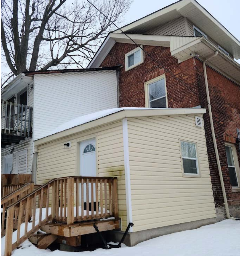
Figure 1: View of the existing rear mudroom at 523 Johnson Street. The proposed second storey addition, containing a new bedroom, would be placed directly above the mudroom. This will mirror the rear addition of the neighbouring unit, but without a balcony.
