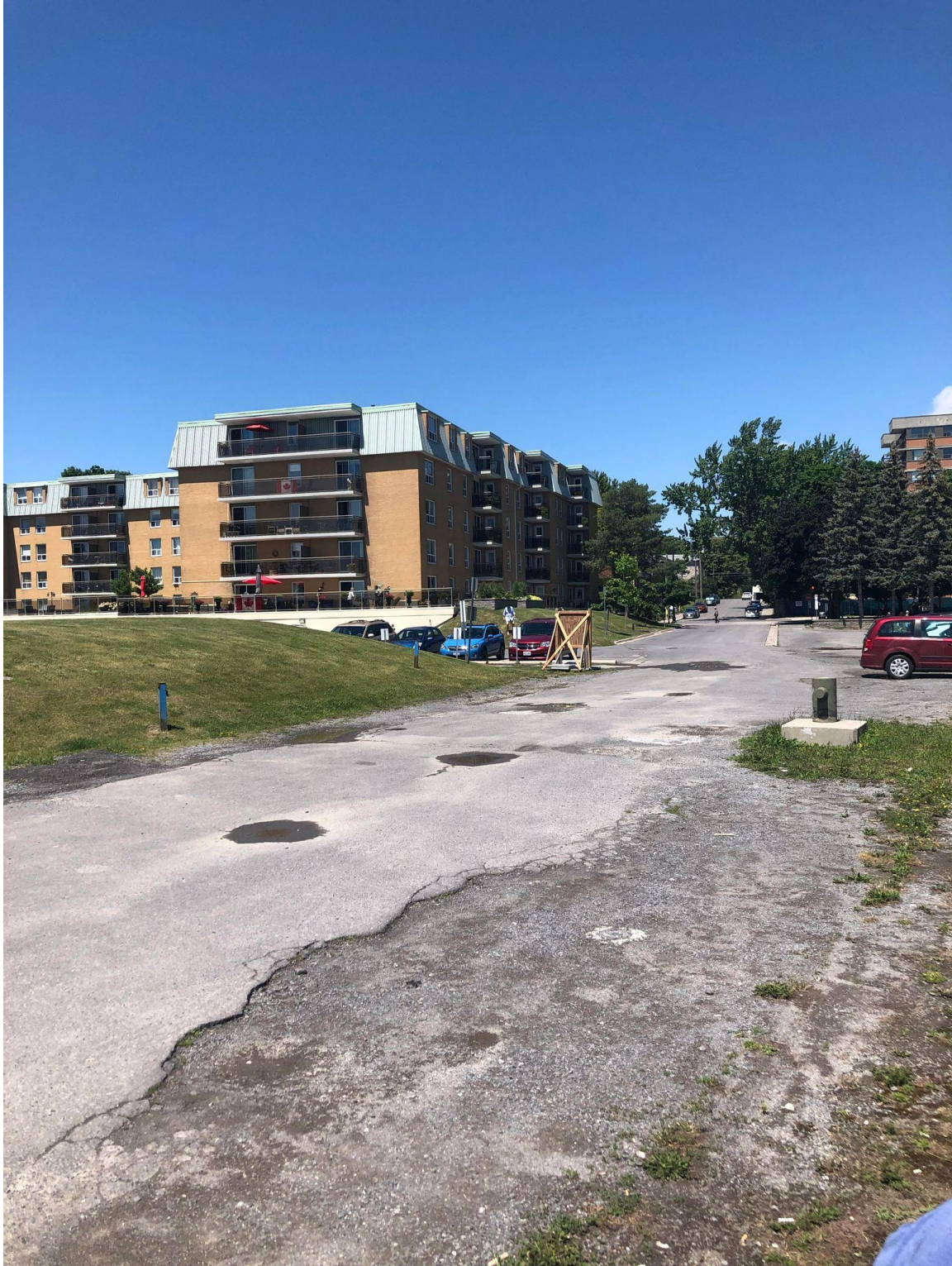
View from fencing on-site west towards Shipyards building
