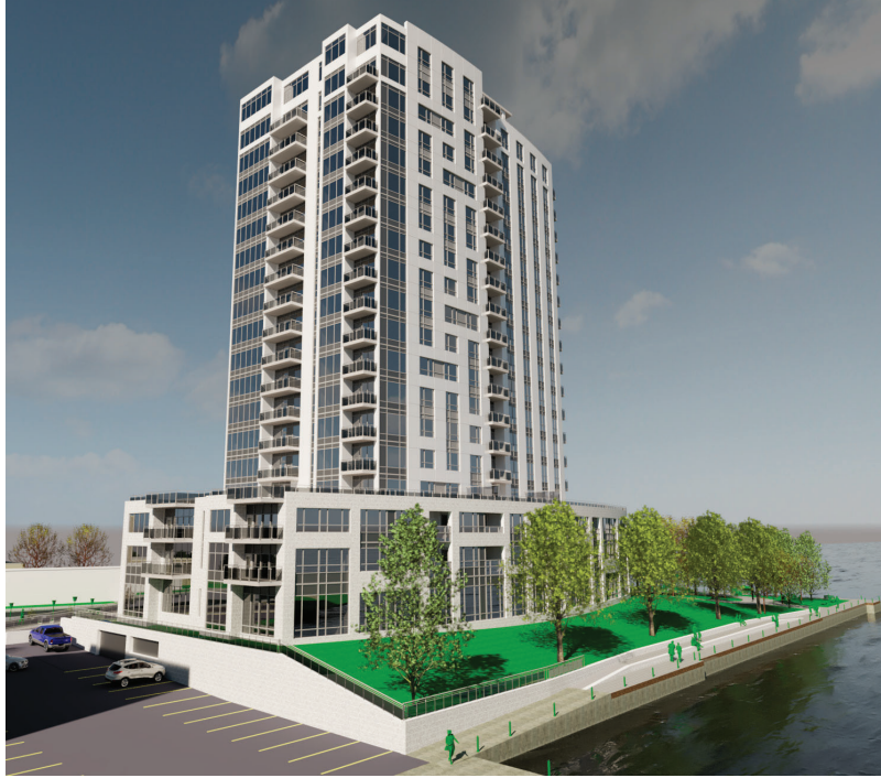
Rendering of the proposed tower, aerial view looking south-east (Alexander Wilson Architects, 2023).
