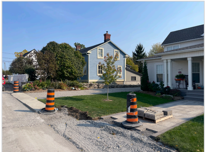
Figure 6: Looking east along Wellington Street from the frontage of the subject property.
