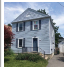
EXISTING FRONT ELEVATION IMAGE
