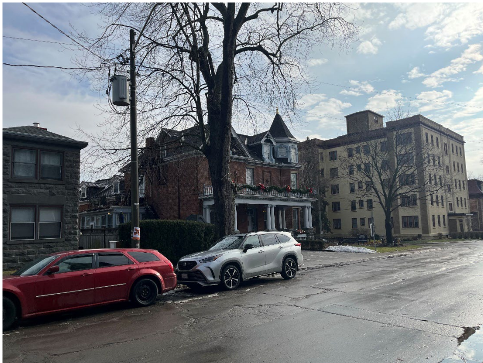
Figure 4: Subject property, as viewed from Sydenham Street.
