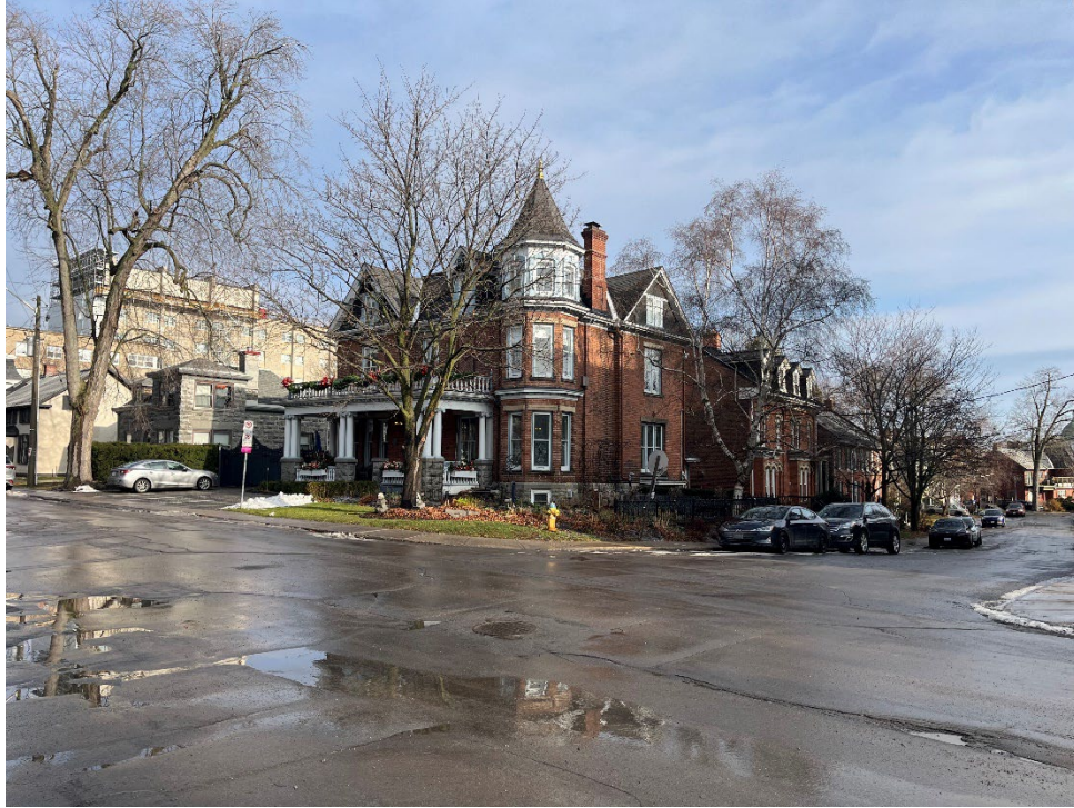
Figure 3: Subject property, as viewed from Sydenham and William Street intersection.
