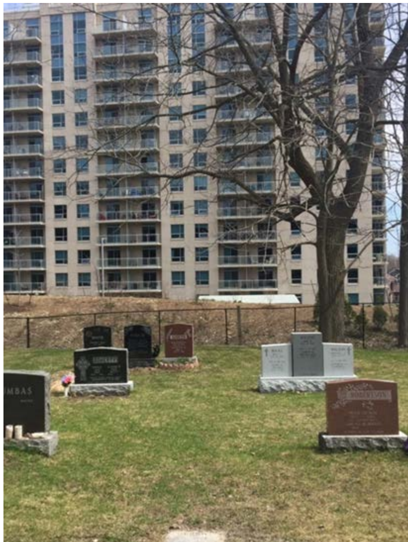
View towards tower 1 May 2020
