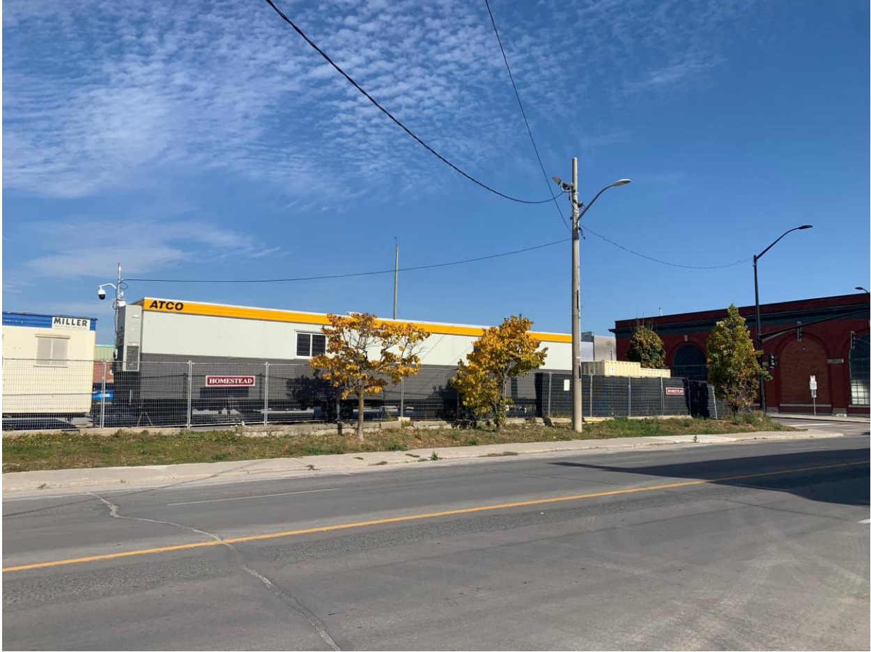
Figure 2: Front facing view of the subject property taken from the Queen Street frontage (October 22, 2024).
