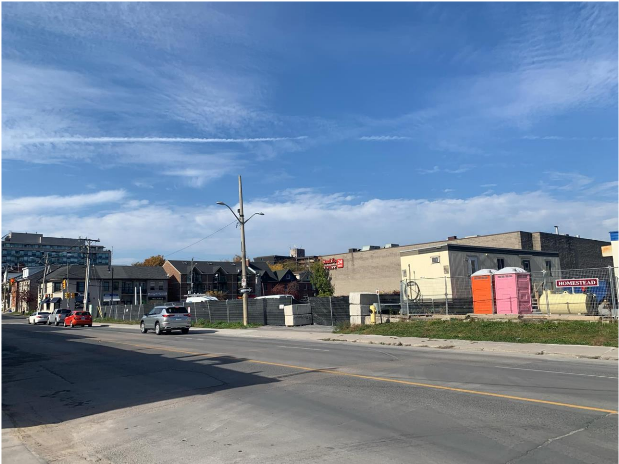
Figure 1: Front facing view of the of the subject property at 55 Queen Street, taken from the Queen Street frontage (October 22, 2024).
