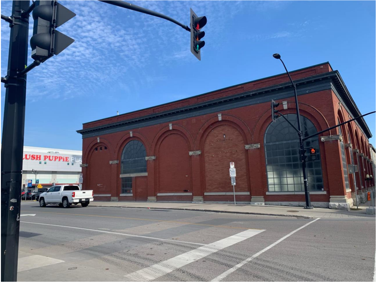
Figure 7: Existing property located across King Street East frontage at 29 Queen Street (October 22, 2024).
