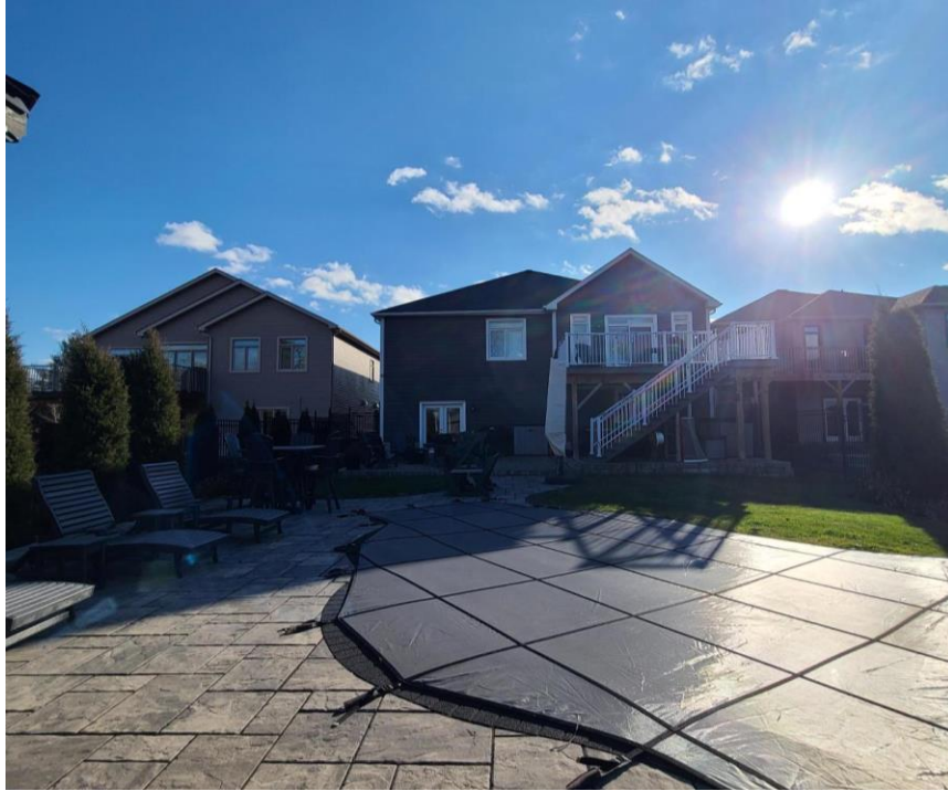
Figure 1- View of home from rear yard of subject property, showing existing deck and area where deck extension is proposed.
