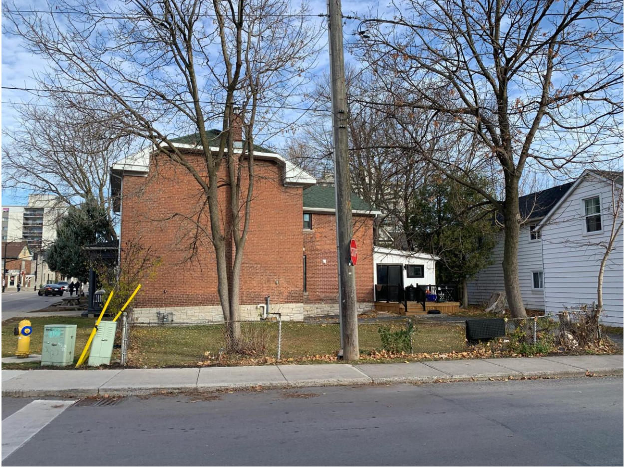
Figure 10: View of the subject property and existing conditions along the William Street frontage, taken on the south side of William Street (November 25, 2024).
