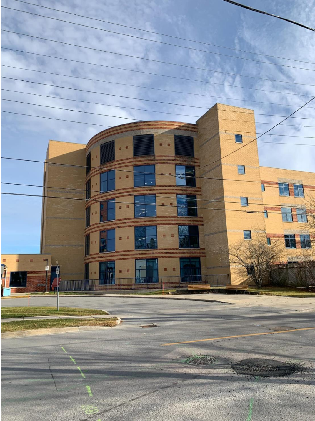
Figure 8: Existing built form of adjacent property at 175 Rideau Street (November 25, 2024).
