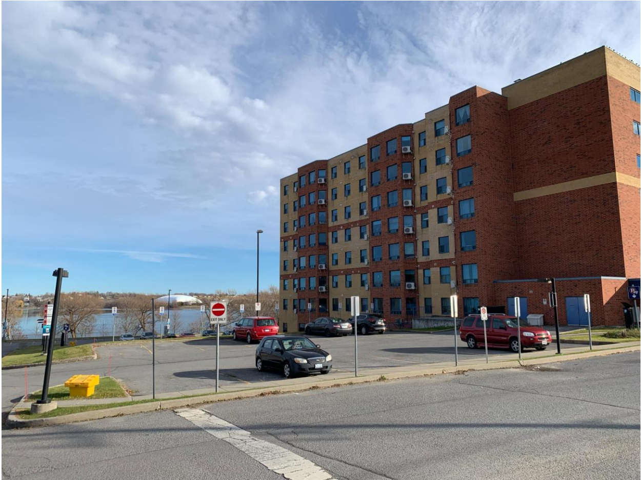
Figure 3: Southeast facing view of the existing 8 storey apartment building, parking area, and downward slope located on the subject property (November 25, 2024).
