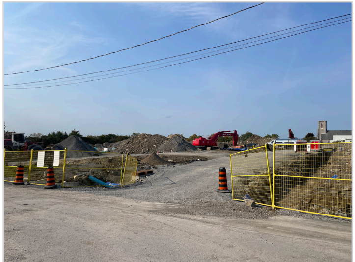
Figure 4: Subdivision under construction north of the subject property across Wellington Street.
