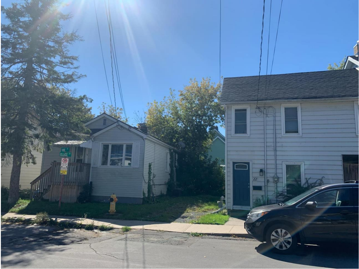
Figure 4: Existing built form directly adjacent and located east of the subject property addressed as 14 Ellice Street (September 26, 2024).
