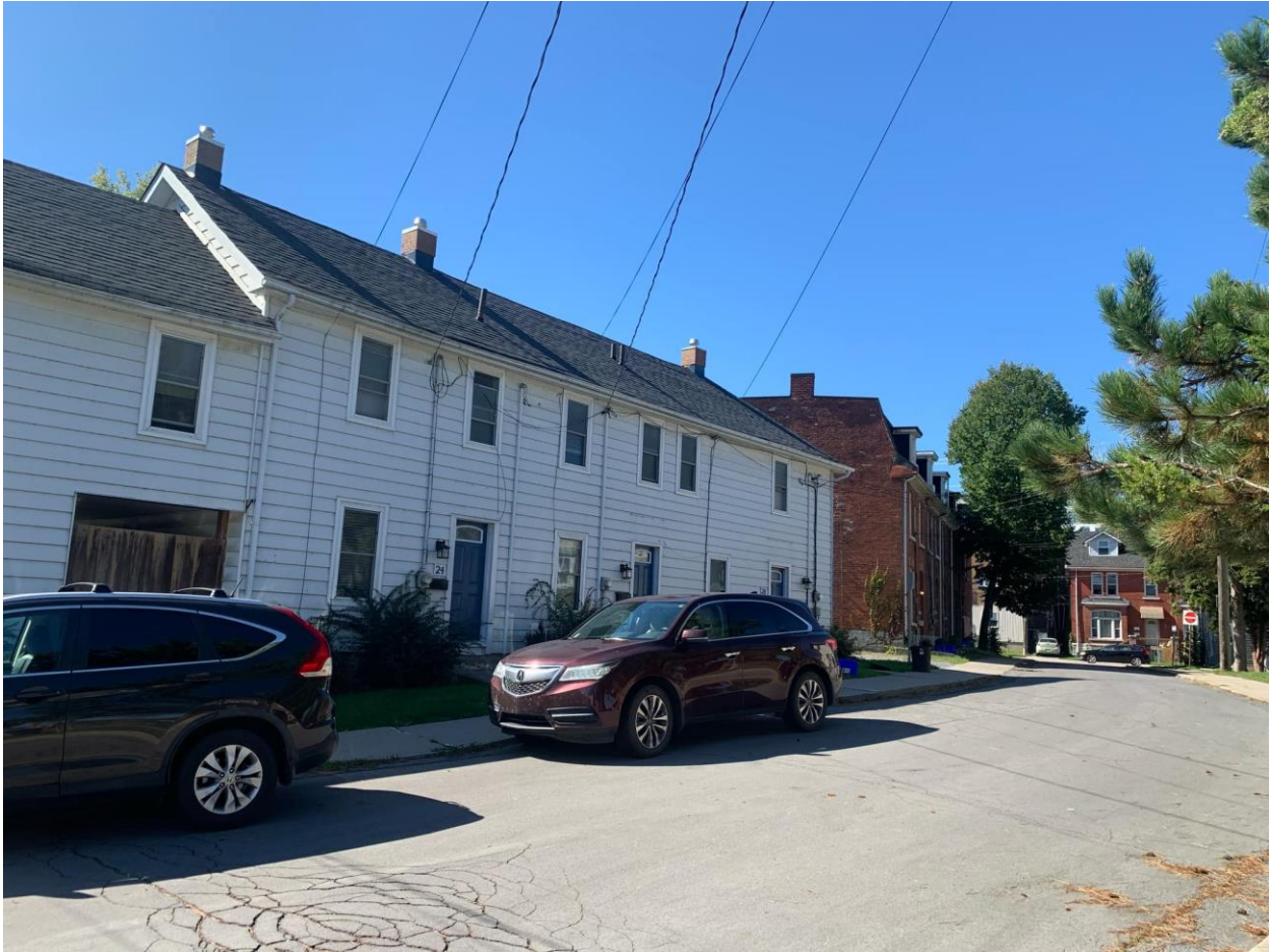
Figure 1: Front facing view of the of the subject property at 22-28 Ellice Street, taken from the north side of Ellice Street (September 26, 2024).
