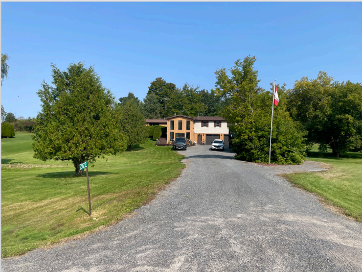
Figure 3: Adjacent property to the east of the subject property.
