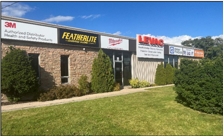
Figure 2: Photo of 25 Railway Street principal building frontage
