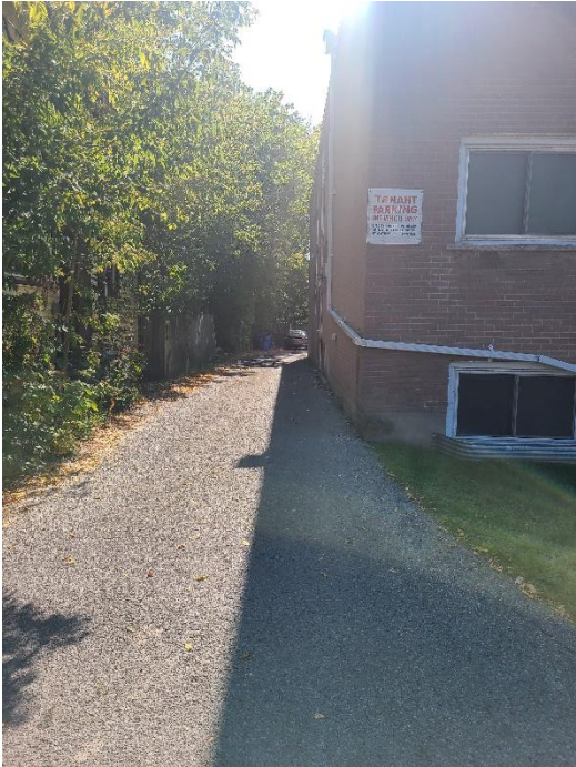
Figure 5- Existing driveway on east side of existing building.
