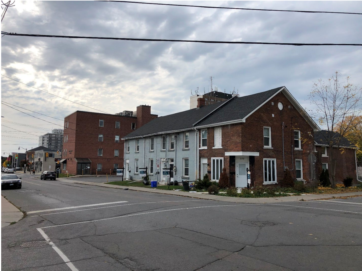
Figure 4: View from the intersection of Barrie Street and Colborne Street, looking southwest. The proposed building would wrap around the rear of the rowhouses pictured in the foreground.
