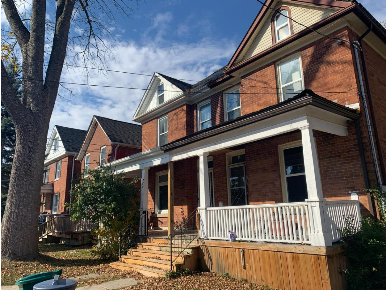
Figure 14: Examples of various built forms found along Birch Avenue, northeast of the subject lands (October 22, 2024).
