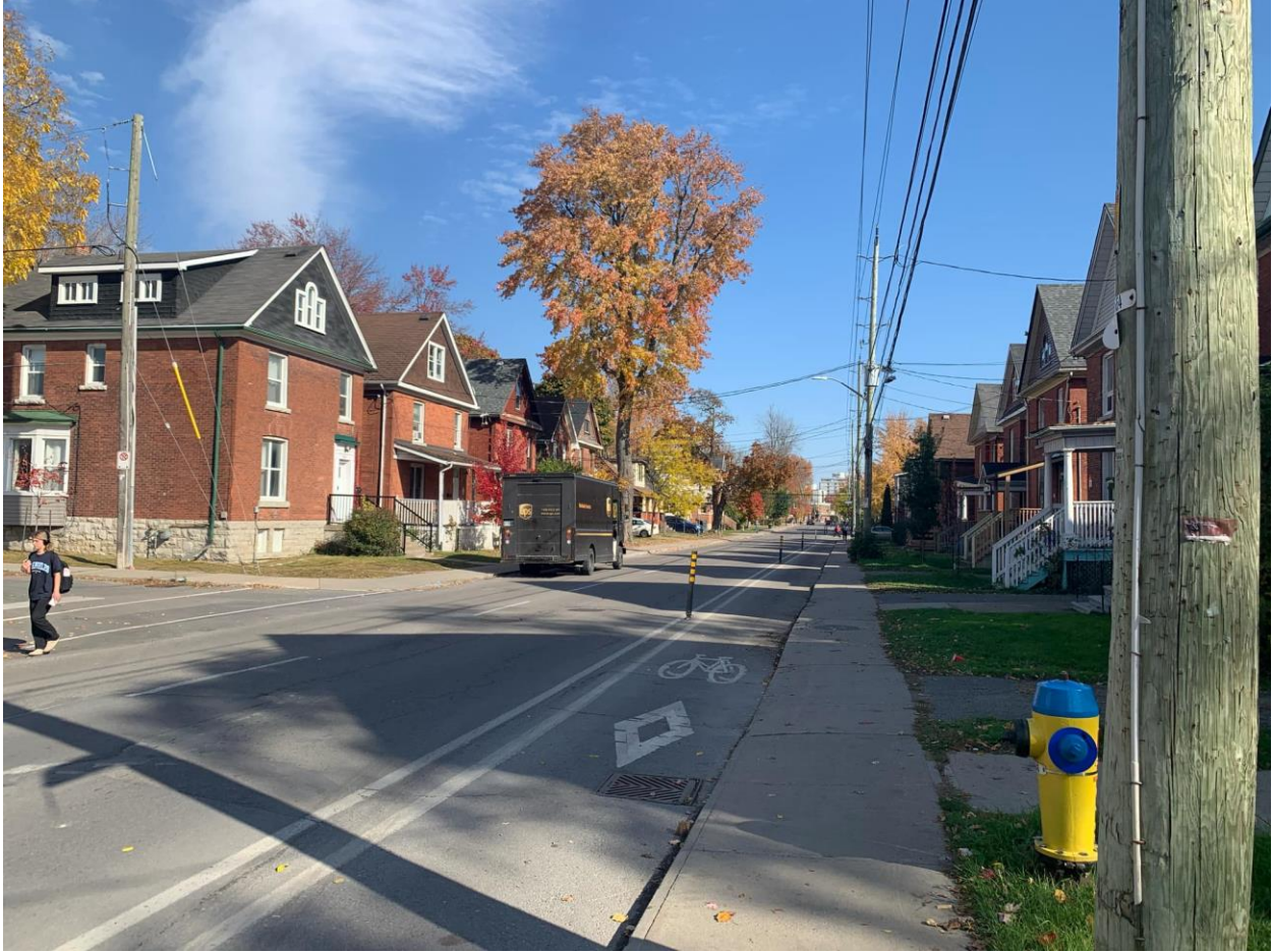
Figure 13: East facing view of the existing bike lanes located on Johnson Street, within walking distance of the subject property (October 22, 2024).
