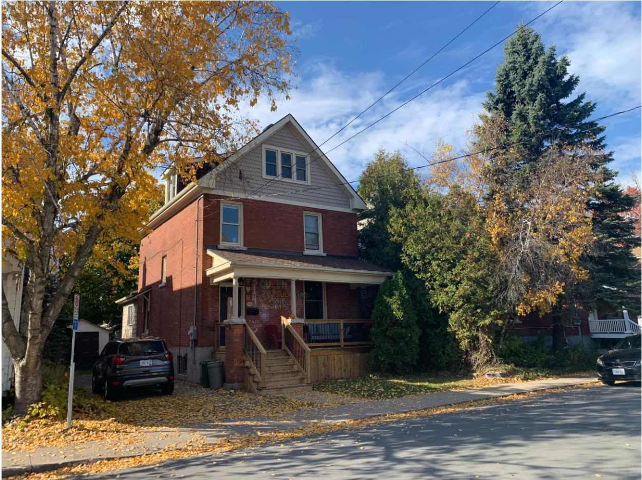
Figure 9: Example of existing built form found along Collingwood Street, addressed as 314 Collingwood Street, located northwest of the subject lands (October 22, 2024).
