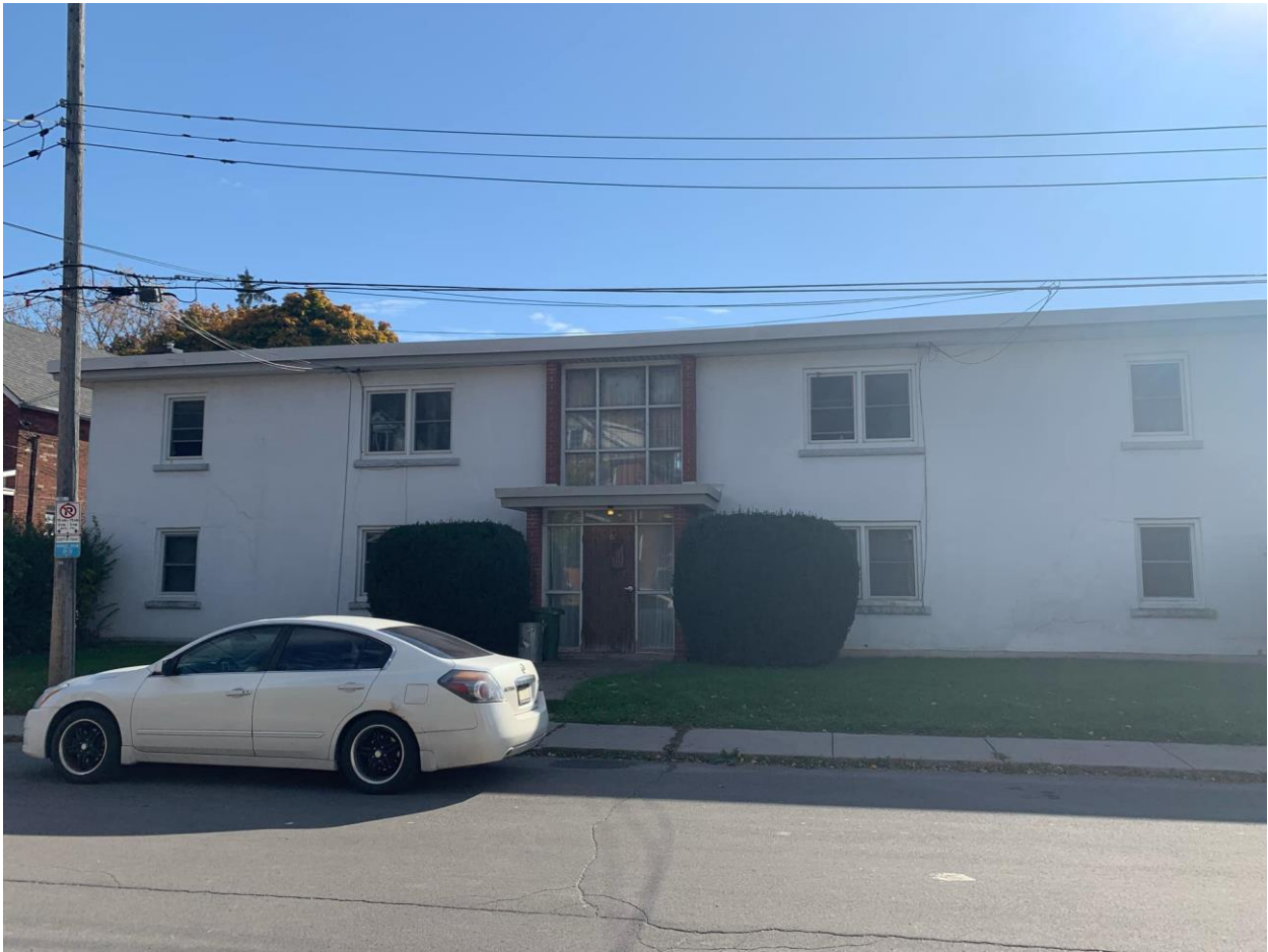
Figure 1: Front facing view of the existing legal non-conforming two-storey four-unit apartment building on the subject property at 10 Birch Avenue (October 22, 2024).
