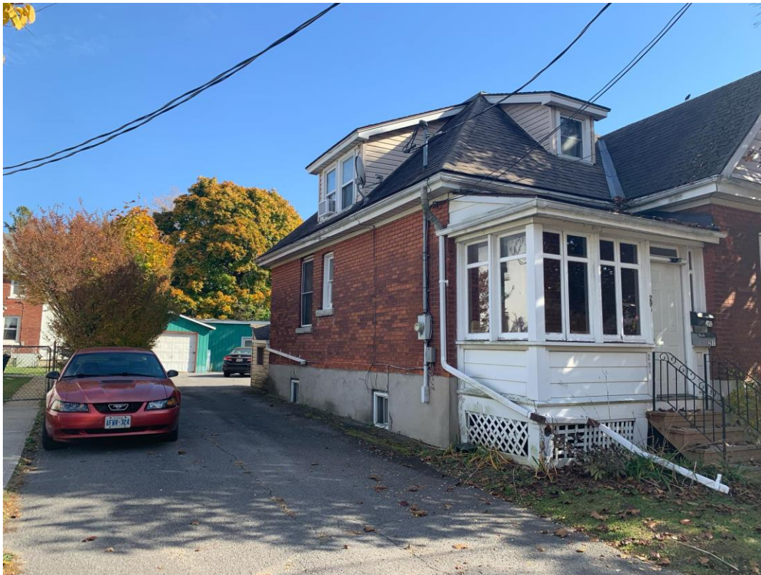
Figure 7: Adjacent property to the south located at 291 Collingwood Street (October 22, 2024)
