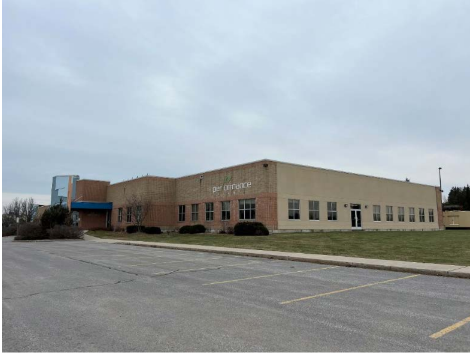
Figure 1: View of the existing building at 1287 Gardiners Road.
