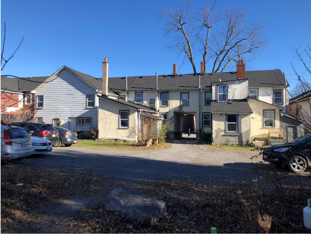
Figure 3: Backyard and rear elevation of existing townhouse.
