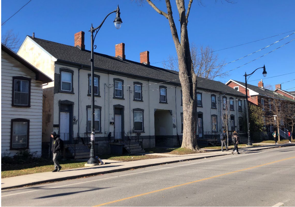
Figure 1: Front elevation of heritage townhouses at 234-242 University Avenue.
