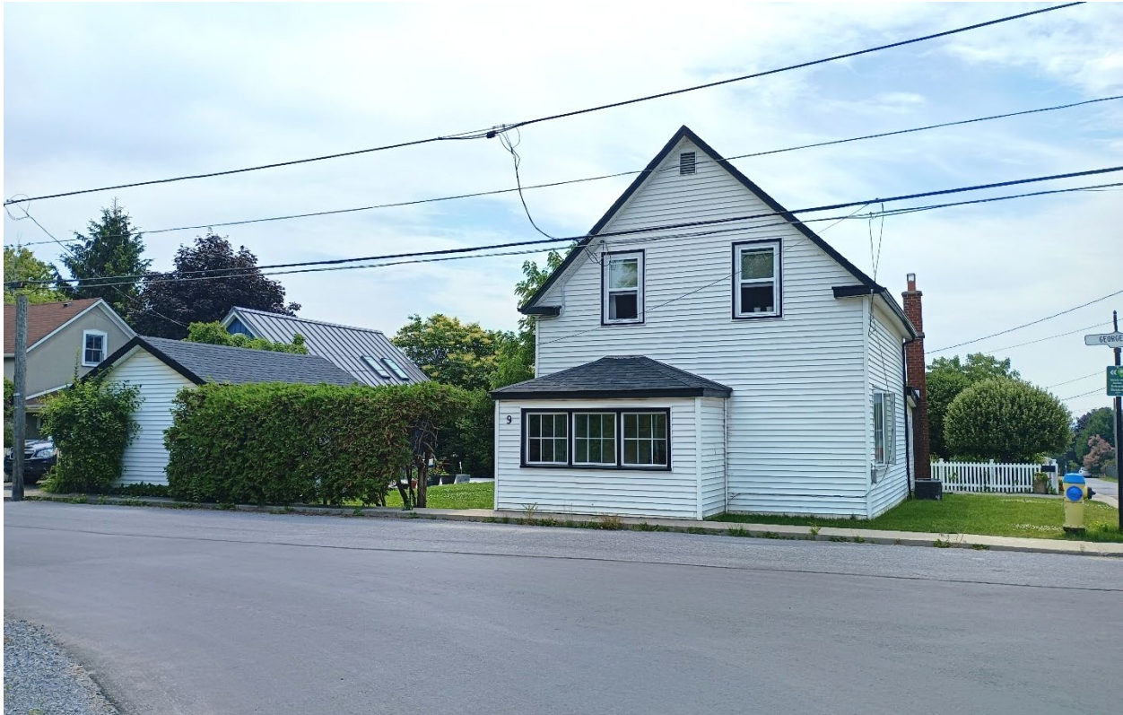
Figure 11: East elevation and setting, June 2024.
