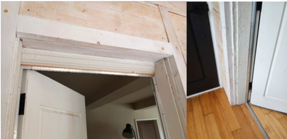
Figure 15: Evidence of original front door trim on George Street entrance, June 2024.
