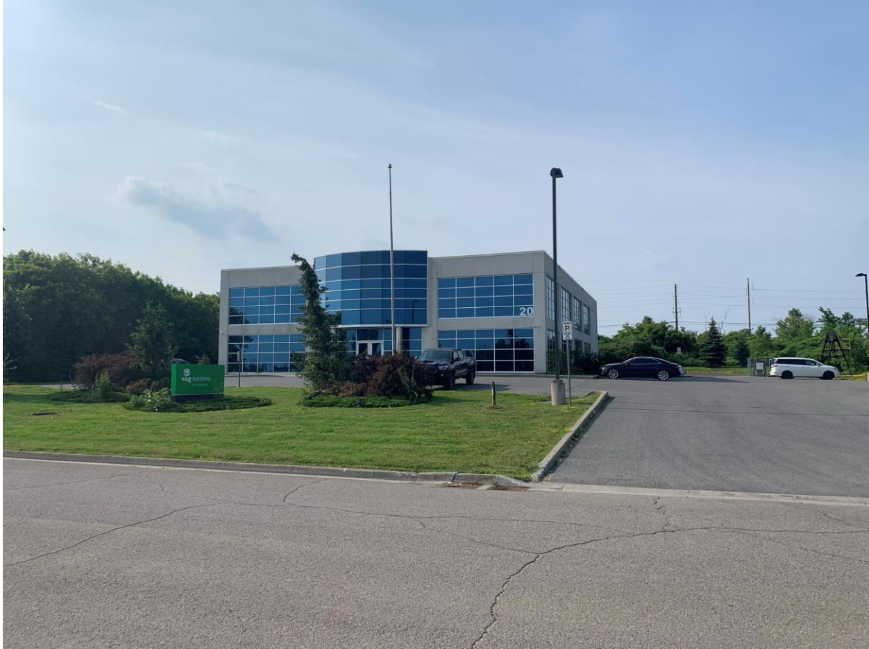
Figure 14. Existing building addressed as 20 Hyperion Court located west of the subject property currently occupied by ESG Solutions (photo taken June 18, 2024).
