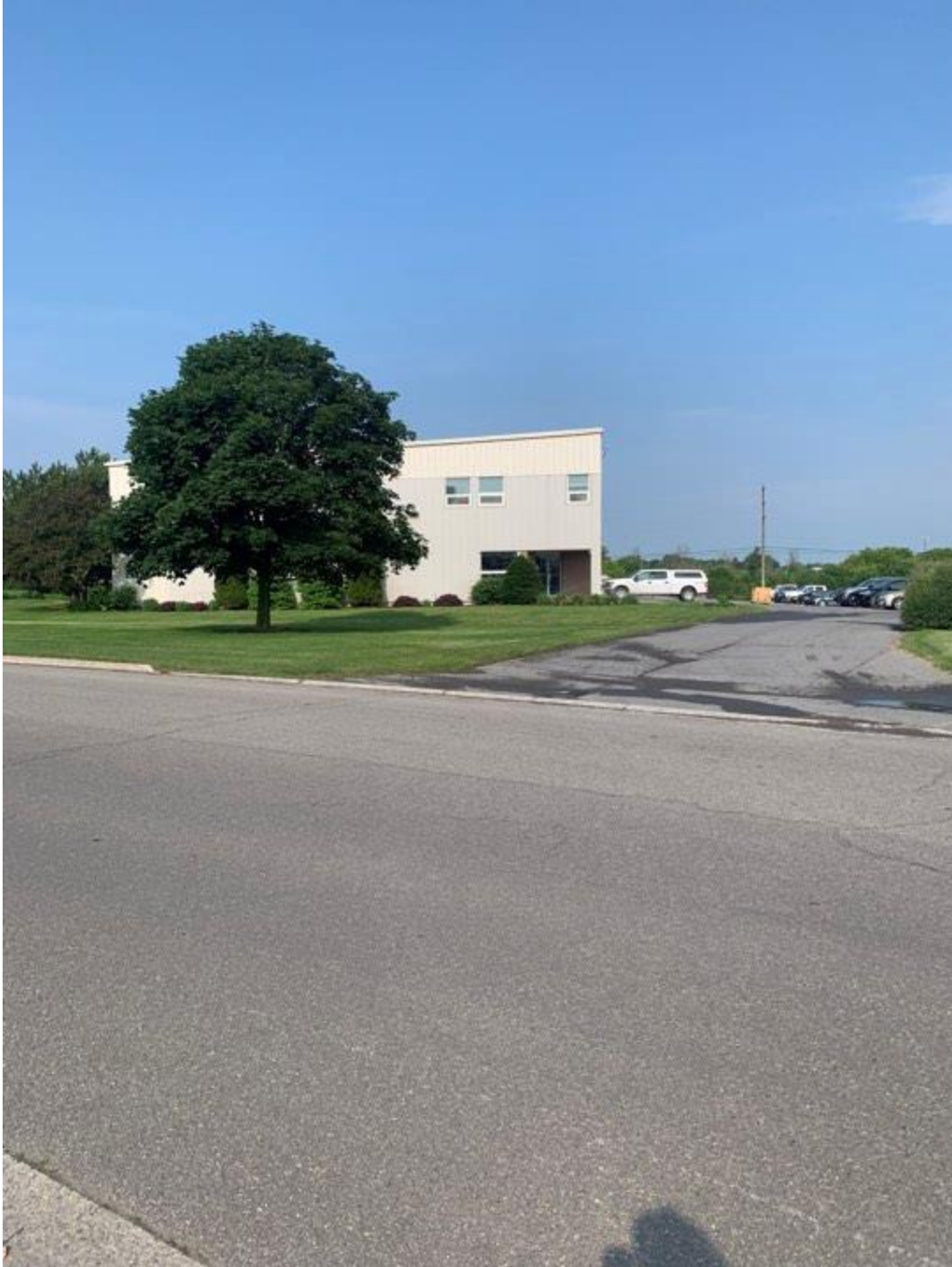
Figure 13. Existing building addressed as 26 Lappan's Lane located west of the subject property with Daltco Electric as the current occupant (photo taken June 18, 2024).
