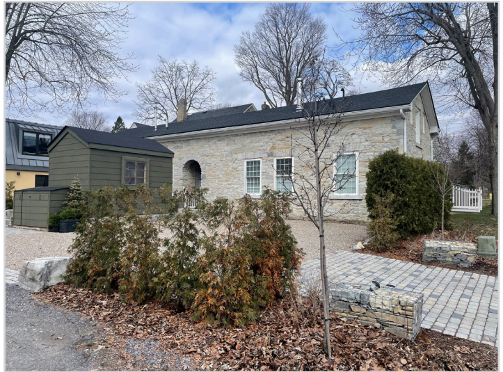
Figure 2: Looking northwest at the shed adjacent to the existing accessory structure to the north.
