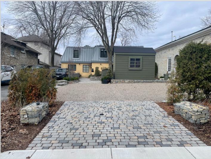
Figure 1: Looking west at the accessory structure on the subject property.
