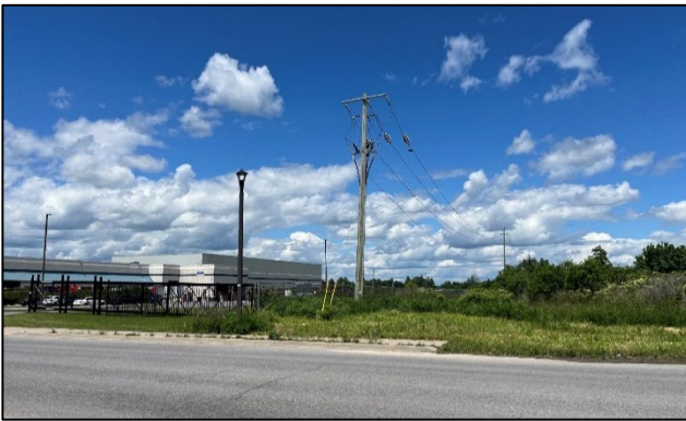
Figure 3: View of east adjacent City owned lands and hydro corridor.
