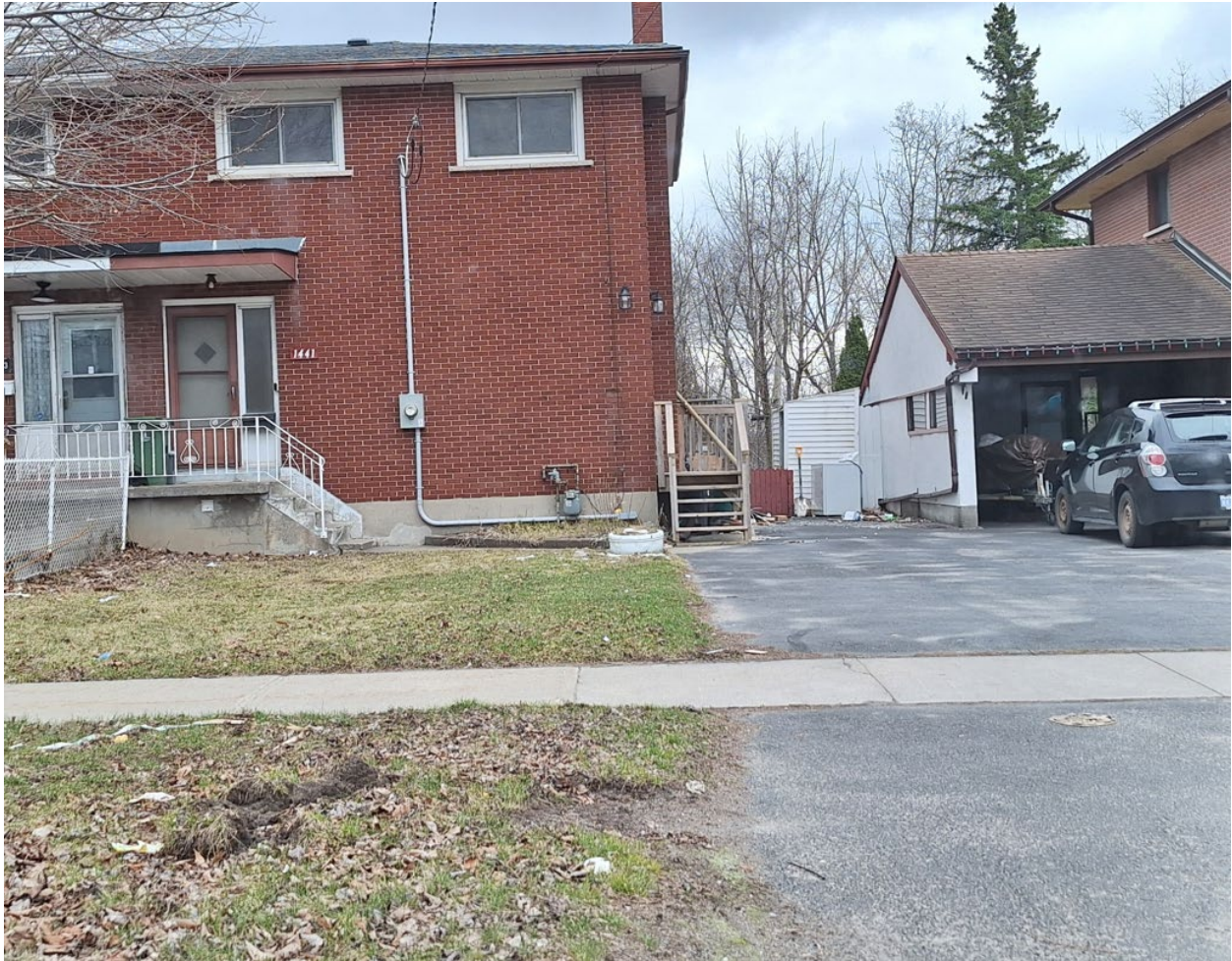
Site Photo – 1441 Montreal Street
