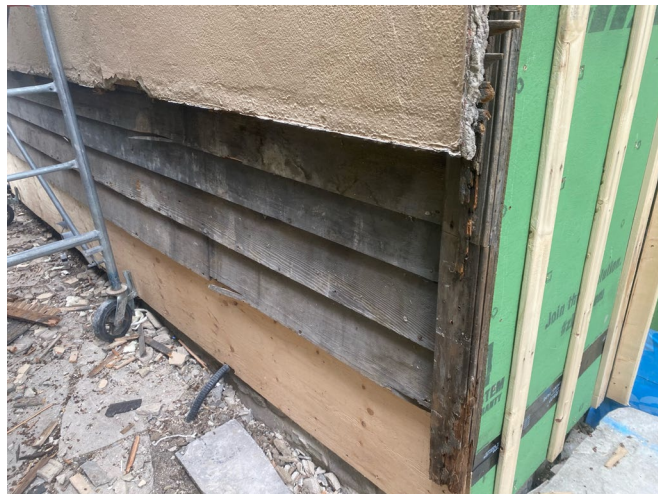
Figures 3 & 4: What is believed to be the original wooden clapboard (rear elevation) and corner trim.
