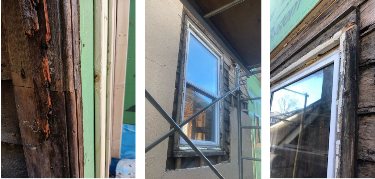
Figures 5, 6 & 7: Detail of original corner trim (note the new piece scarfed into match) and original window trim exposed showing bead detail and small drip moulding.
