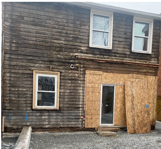
Figures 3 & 4: What is believed to be the original wooden clapboard (rear elevation) and corner trim.
