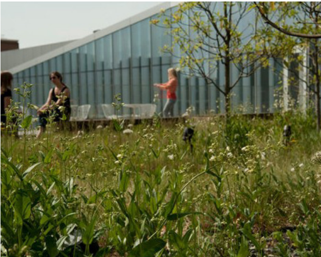
All: Green roofs as an effective way to filter and retain stormwater and potentially create meaningful habitat
