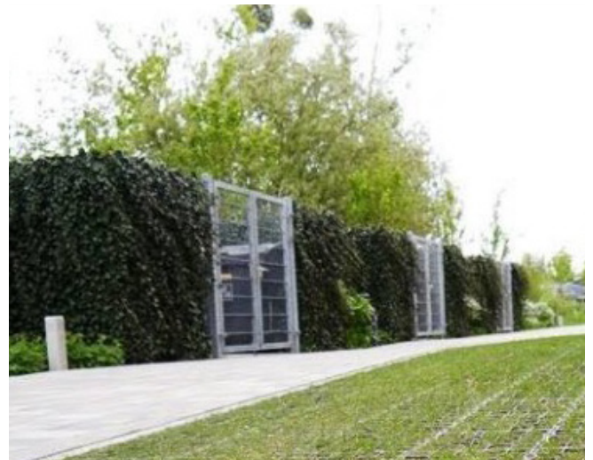
Top: Loading and servicing areas are located away from primary street frontages and visually screened.
