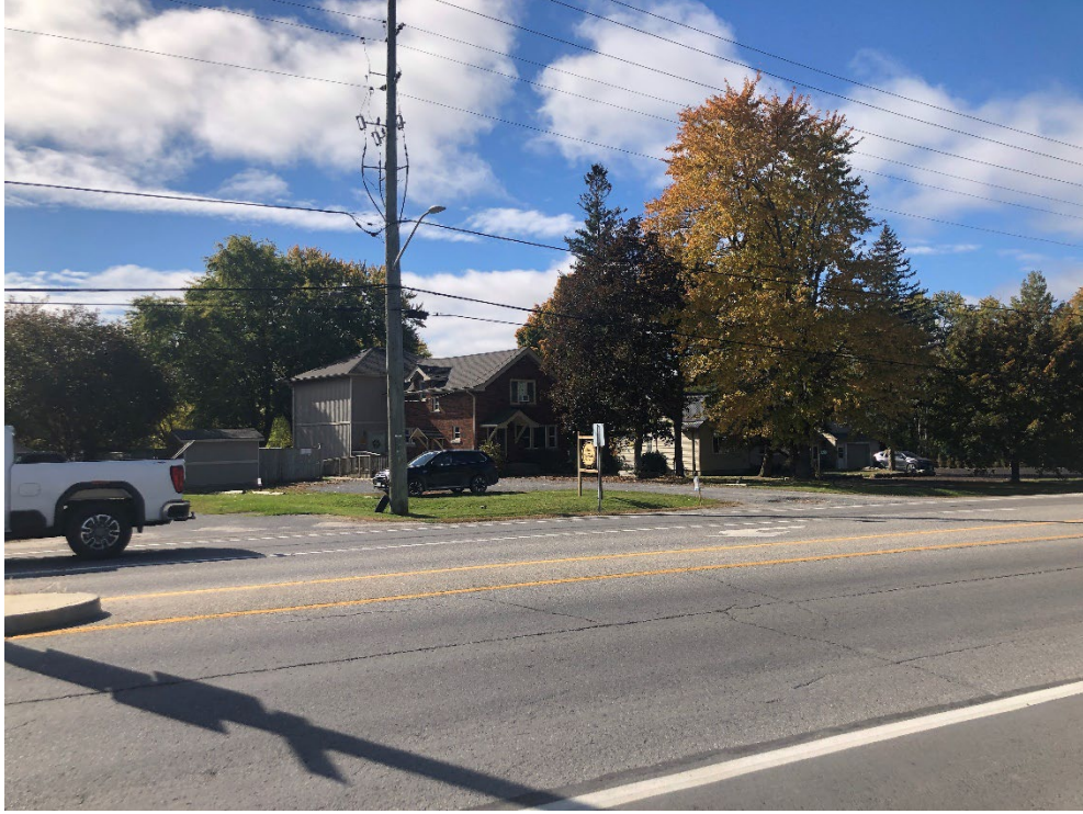
Figure 1: Subject property as viewed from the Woodhaven Drive intersection
