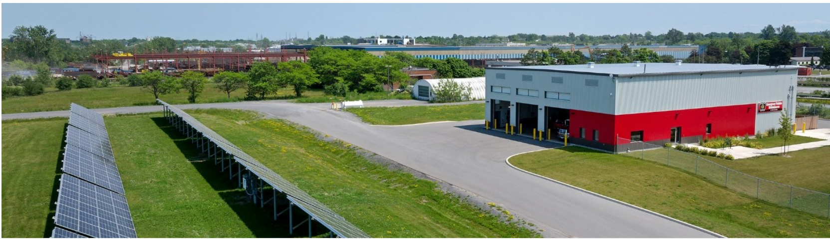
Figure 20. New Kingston Fire & Rescue Maintenance Garage
