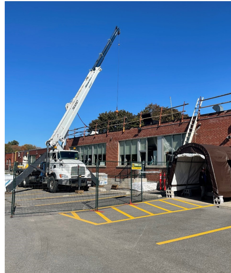
Figure 16. Kingston Senior's Association During Roof Replacement
