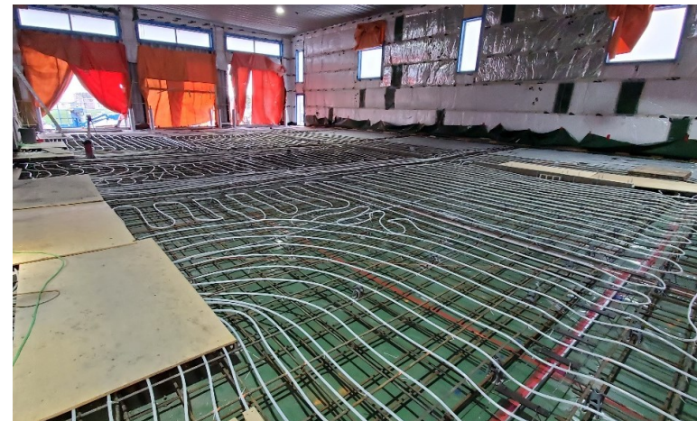
Figure 4. New Fleet Maintenance Garage Under Construction
