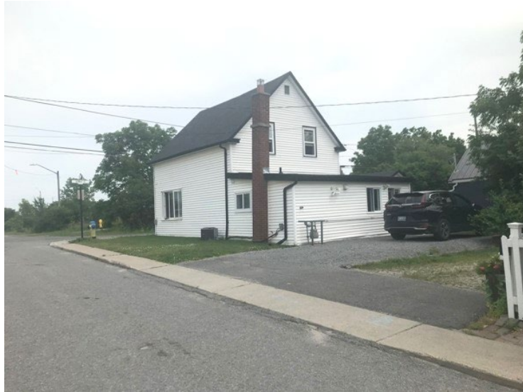
Figure 9: Southwest elevation, June 2024.
