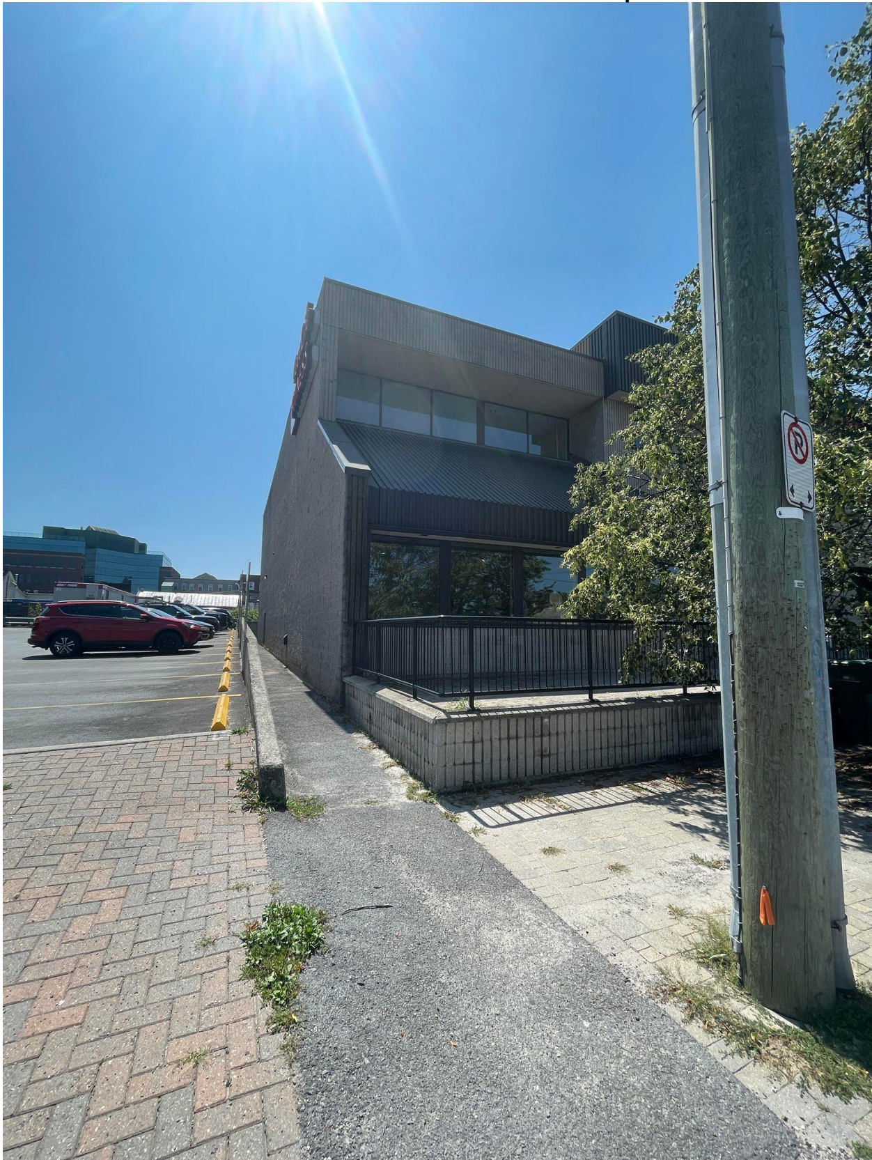
View of existing building face abutting adjacent commercial (LCBO) site
