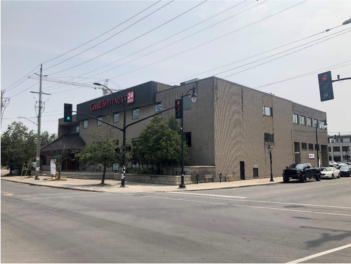
View to corner frontage at Barrack and Wellington Streets
