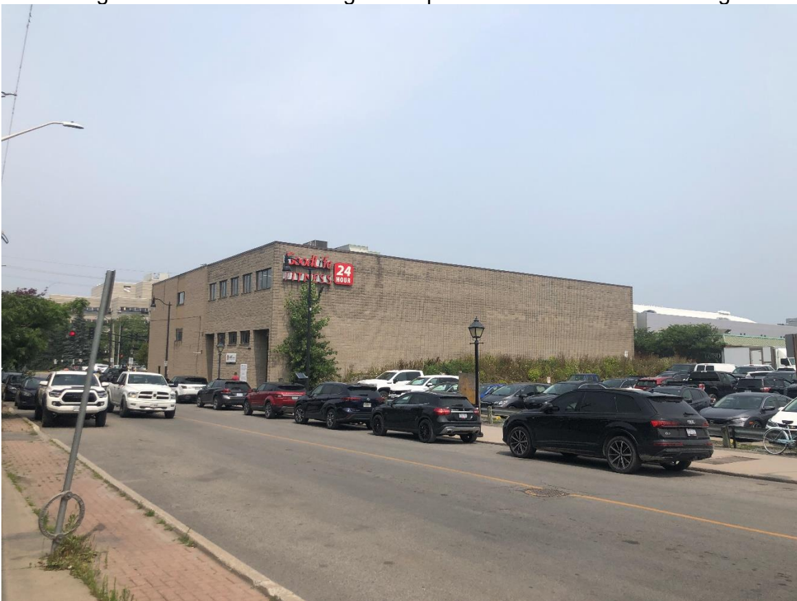
View to site from west sidewalk on Wellington Street
