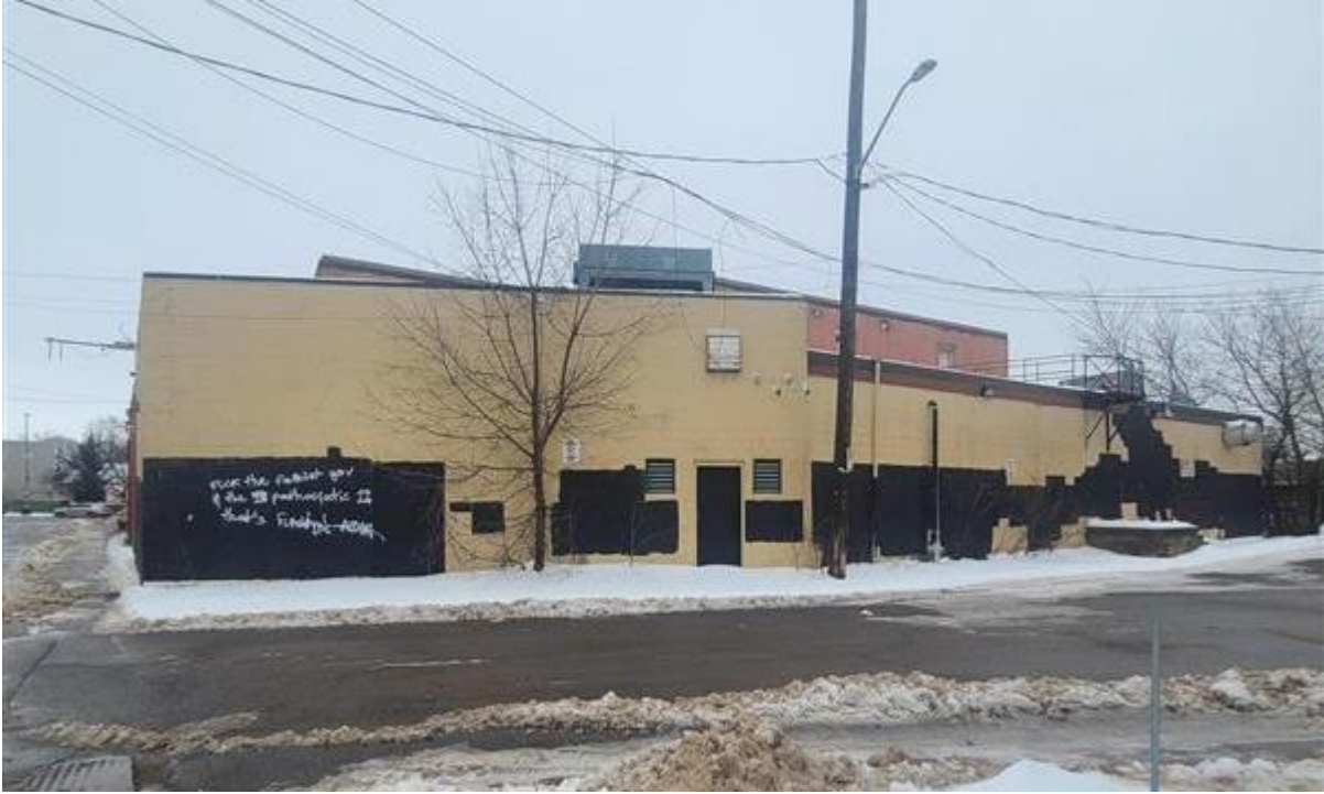
Figure 7: View of 525 Princess Street from the south side of Creighton Street.
