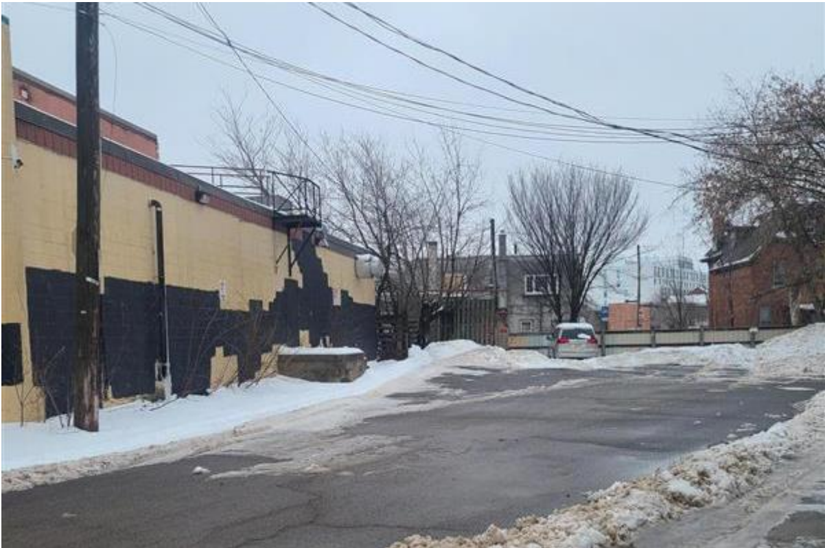
Figure 8: View of Creighton Street with 525 Princess Street on left.
