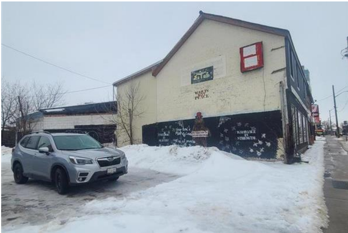
Figure 4: View of existing building addressed 525 Princess Street, currently vacant.
