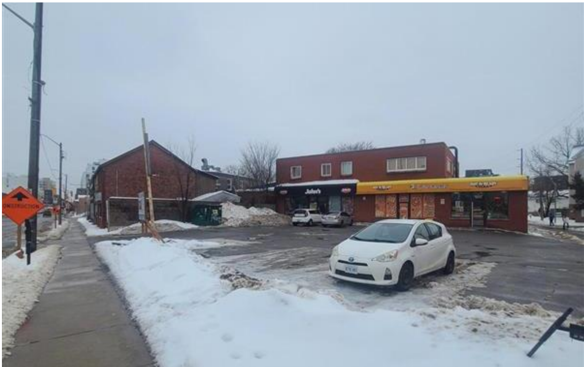
Figure 6: View of 525 Princess Street from the northwest corner of Princess Street and Chatham Street.
